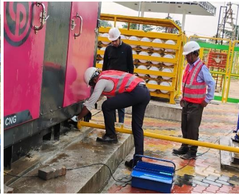
2. Leakage rectification by O&M team.
